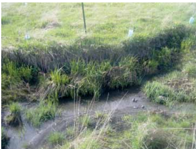
Biolox installed on streambank
