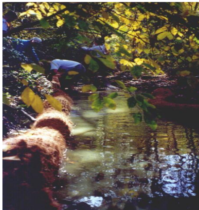
EXAMPLE OF BIOLOGS ANCHORED ALONG A LAKESHORE
